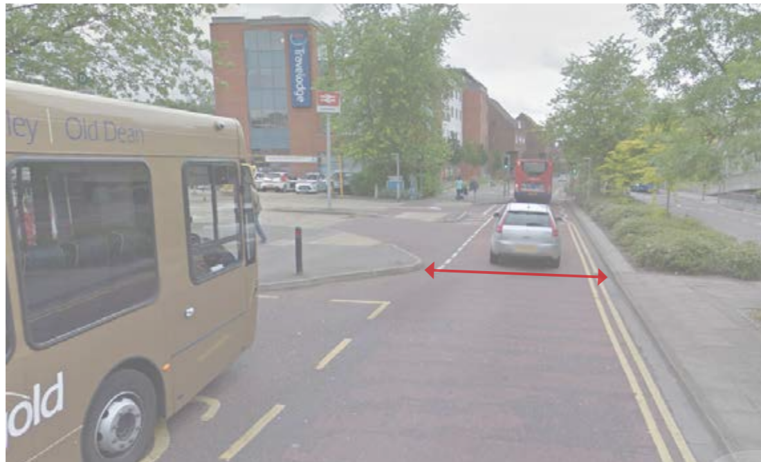
Pinch points along the length of the street reduce the width to a single carriageway at points, buses have to exit and reenter lanes of traffic at these points.
