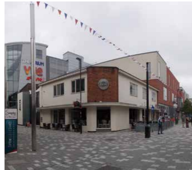
Existing condition - Park Street.
