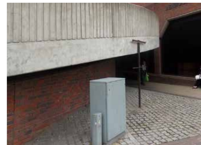
Poor quality pedestrian connections to the station
